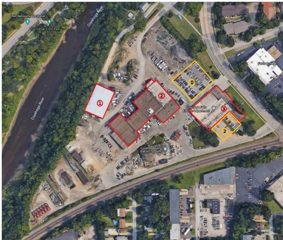
Figure 3: Electric/Service Department – Roof and Parking Lot Potential
