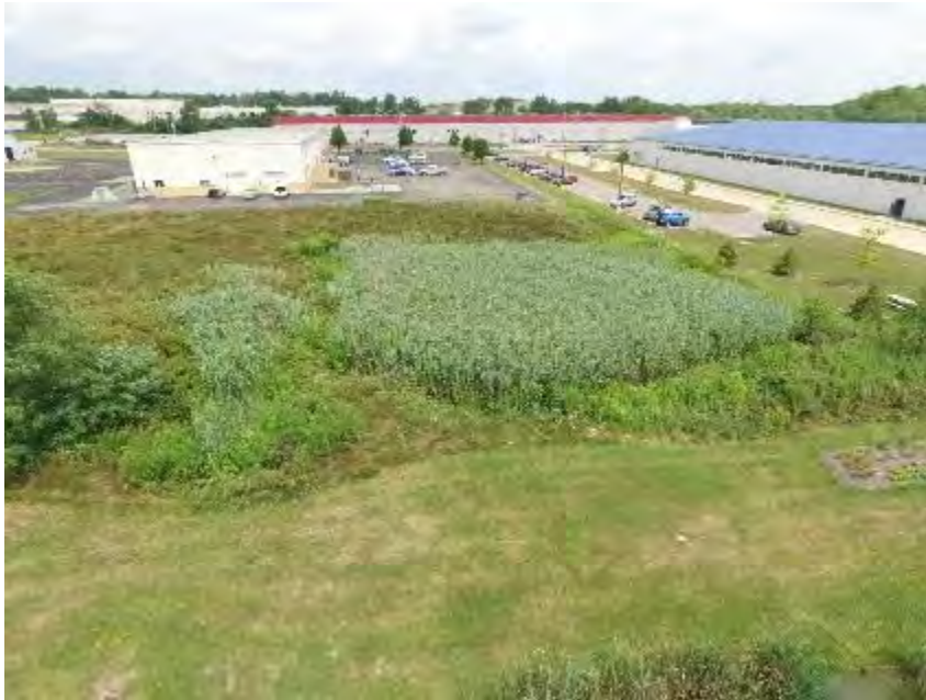
Figure 14. Existing Detention Basin at 120 Marc Dr.
