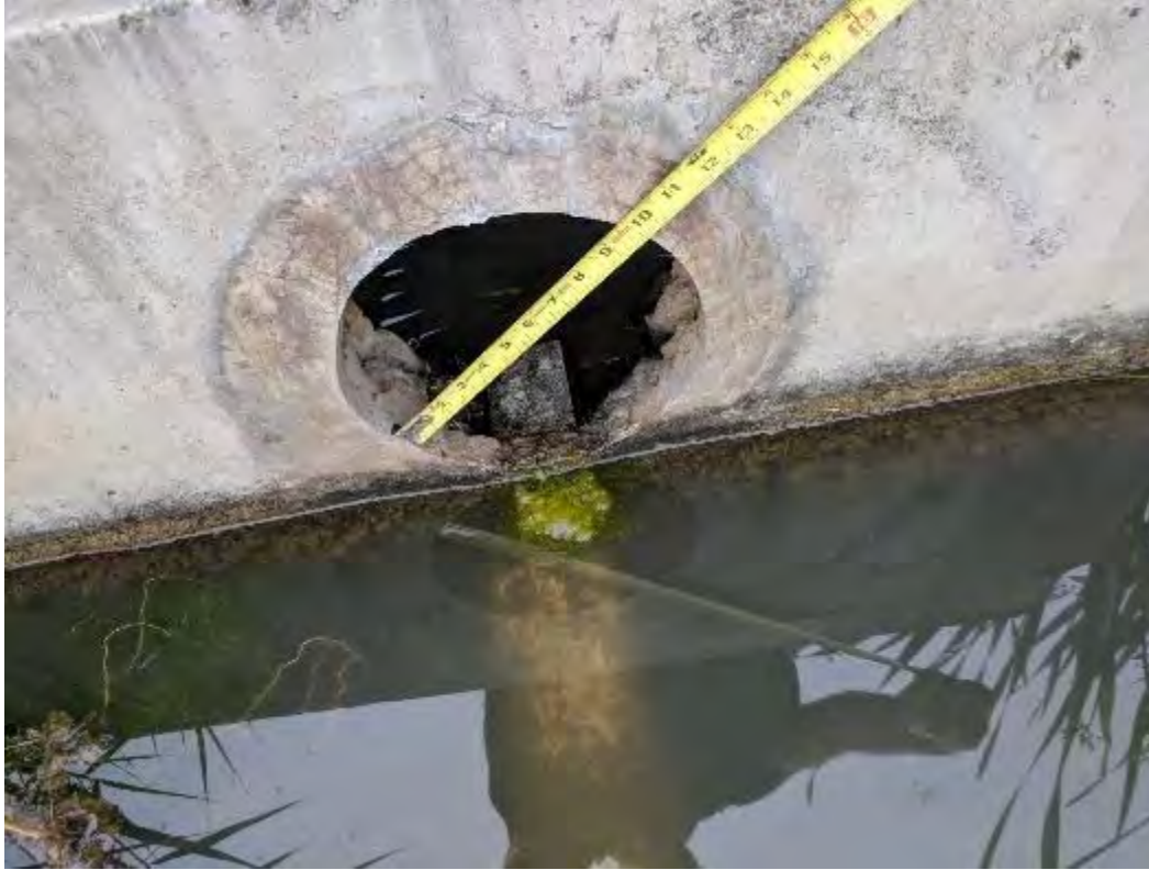
Figure 13. Measuring Detention Orifice Diameter (~9.5 in)
