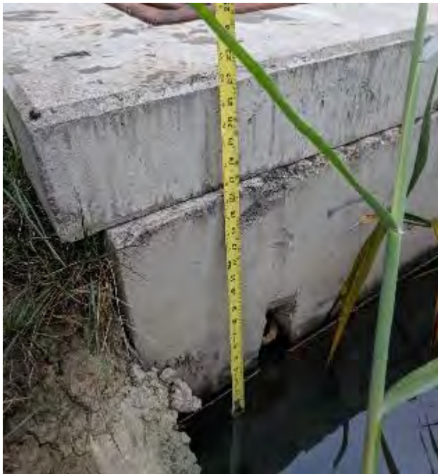
Figure 12. Measuring Elevation Difference (~1.83 ft) between Permanent Pool and Basin Overflow
