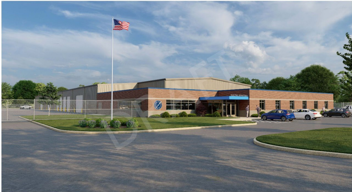
CUYAHOGA FALLS ELECTRIC DEPT.
